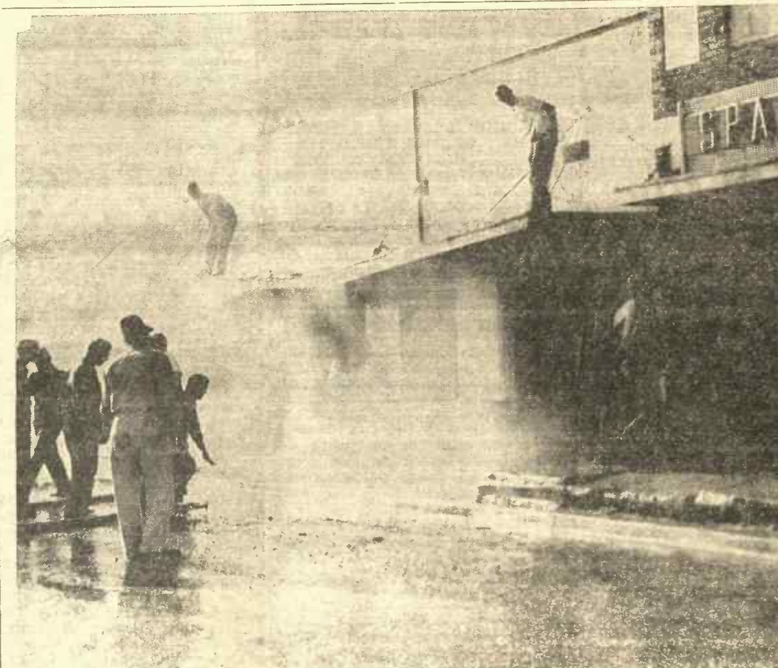
FIRE FIGHTERS AT BELMONT—This view shows a portion of the burning structures and some of the fire fighters who helped to subdue the disastrous blaze Monday that destroyed up to $100,000.00 in property including the Belmont Dollar Store and the Washateria. Porch roof in foreground is in front of Hoyt Griffins auto supply store which was damaged with smoke and water.
